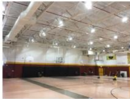
New efficient LED lights
